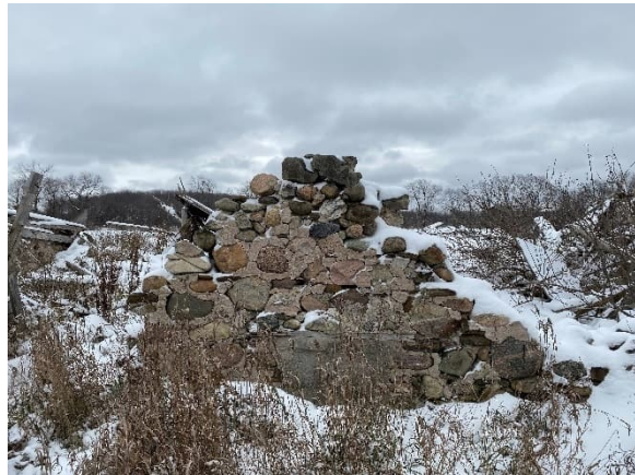
Plate 29: Parged fieldstone walls of Structural Foundation No. 2
