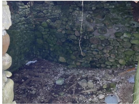
Plate 33: Fieldstone wall of below grade cellar interior
