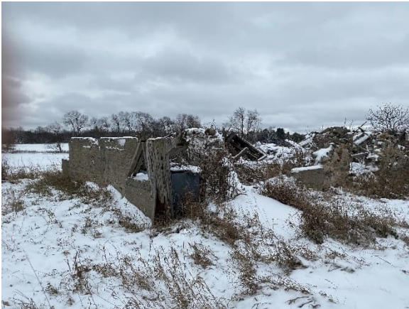
Plate 28: Concrete walls of Structural Foundation No. 2
