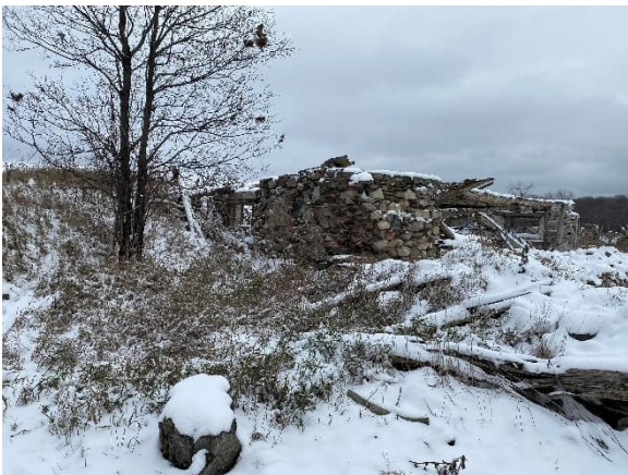
Plate 21: Earthen ramp north of Structural Foundation No. 1
