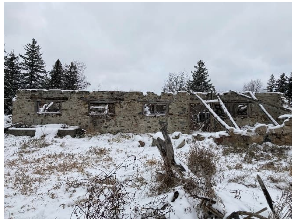
Plate 20: South elevation of Structural Foundation No. 1
