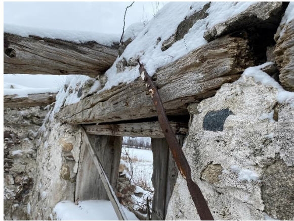
Plate 24: Wood lintel and frame
