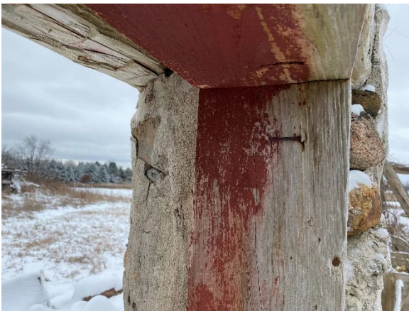
Plate 25: Wood window frame joint
