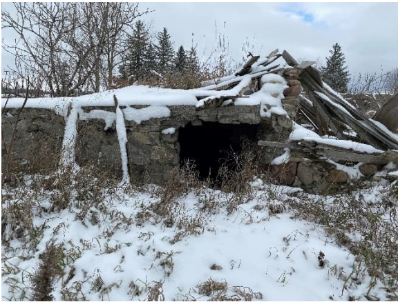
Plate 32: Entrance to below grade cellar
