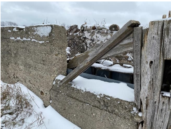
Plate 30: Wood fenestration elements of Structural Foundation No. 2
