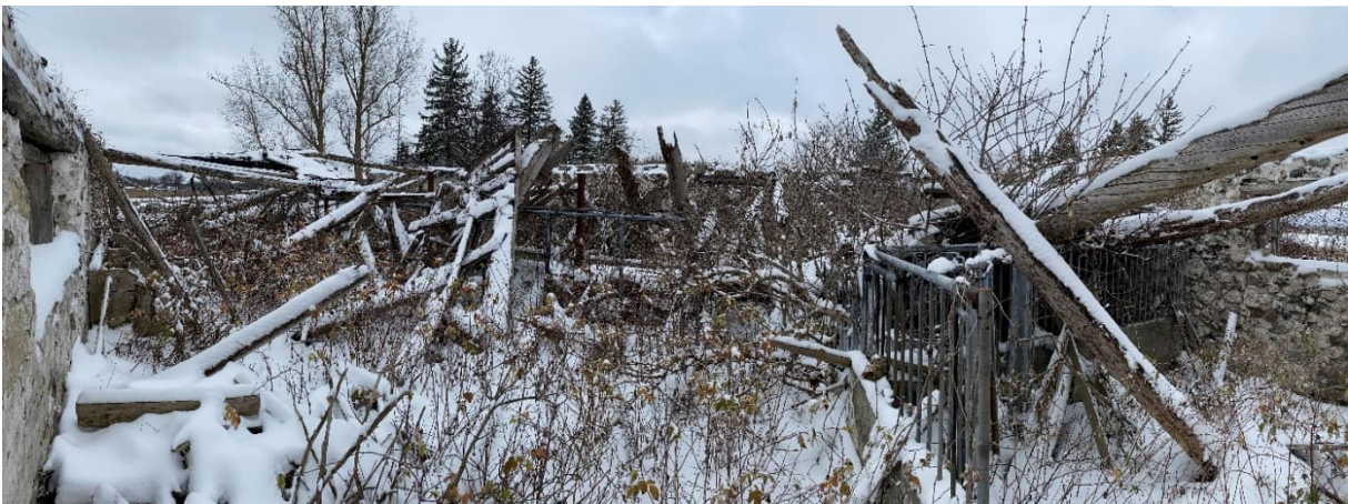
Plate 27: Panoramic photo of Structural Foundation No. 1 interior
