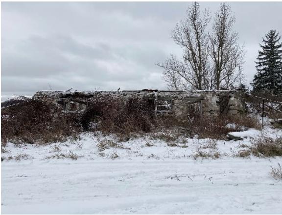
Plate 19: West elevation of Structural Foundation No. 1
