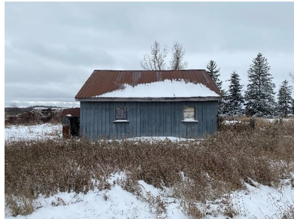
Plate 18: East elevation of outbuilding
