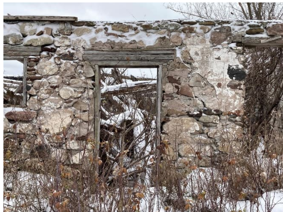
Plate 22: Parged fieldstone wall and doorway
