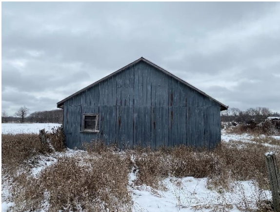
Plate 17: North elevation of outbuilding
